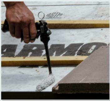
**The Dual Fix Hybrid System** provides the verifiable and proven peace of mind of knowing that the roof system is secure. Whereas with a dual-component tile adhesive installation, it takes post-installation destructive testing or a wind event to determine if the concealed attachment method was mixed properly, installed as prescribed (proper paddy size and placement) or actually exists.
